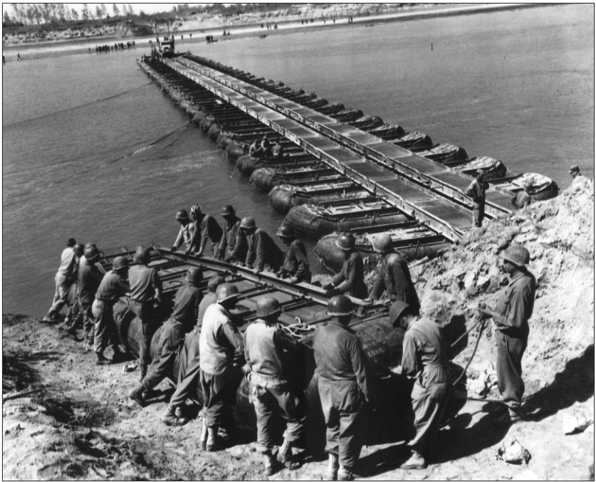
M-2 Treadway Pontoon Bridge under construction across the Po River near Ostiglia (National Archives)
