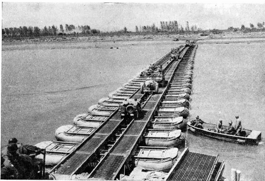
« Engineers toiled to span the swift-running stream with a ponton bridge ».
