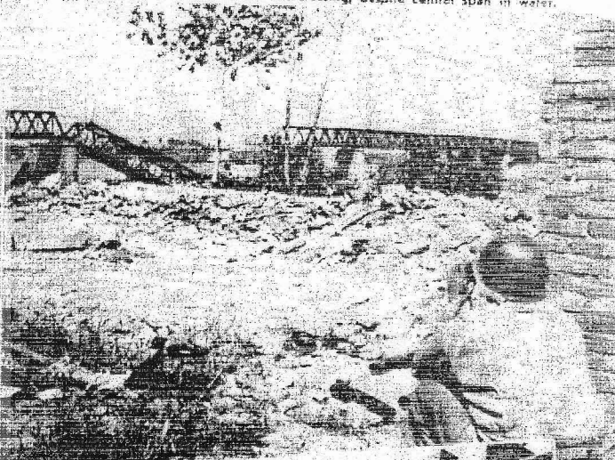
Observer notes extent of damage to iron bridge between Rovere and Ostiglia. Troops of 88th Div. were able to use this crossing, despite central span in water.
