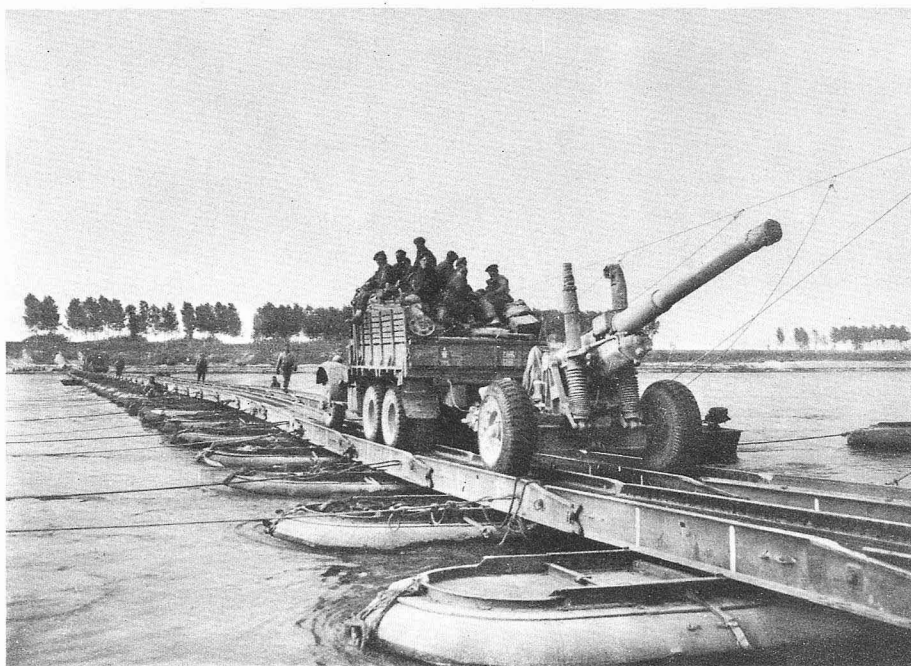
Big guns crossed on a hastily constructed « Floating Treadway ».
