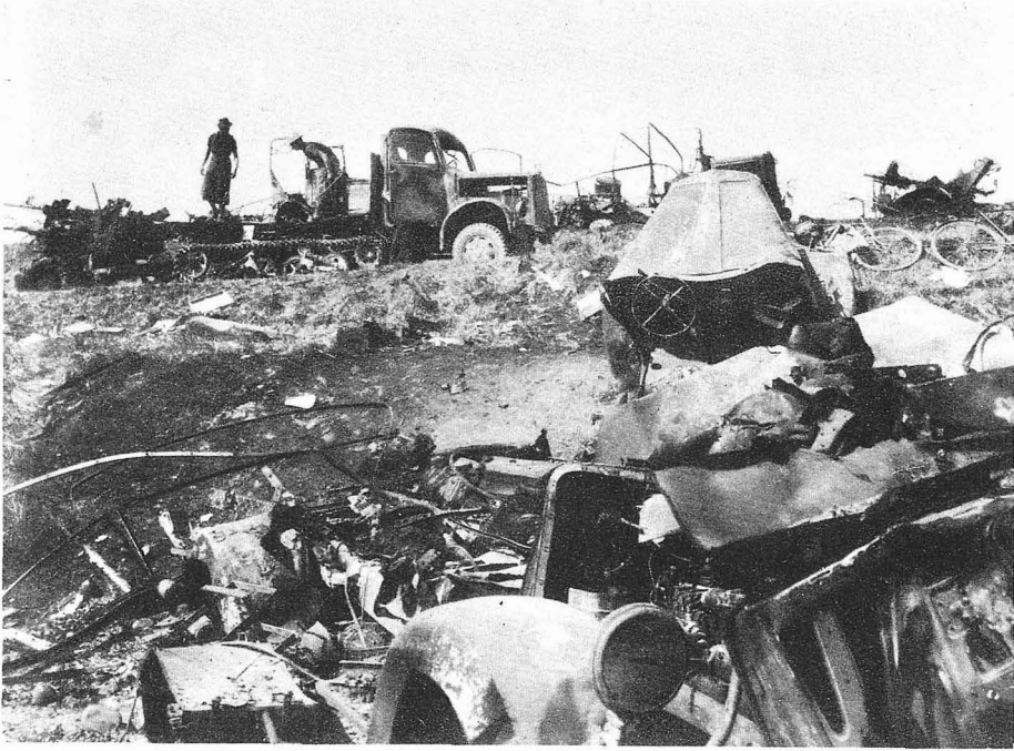
The river bank became a gargantuan junk pile of German equipment.
