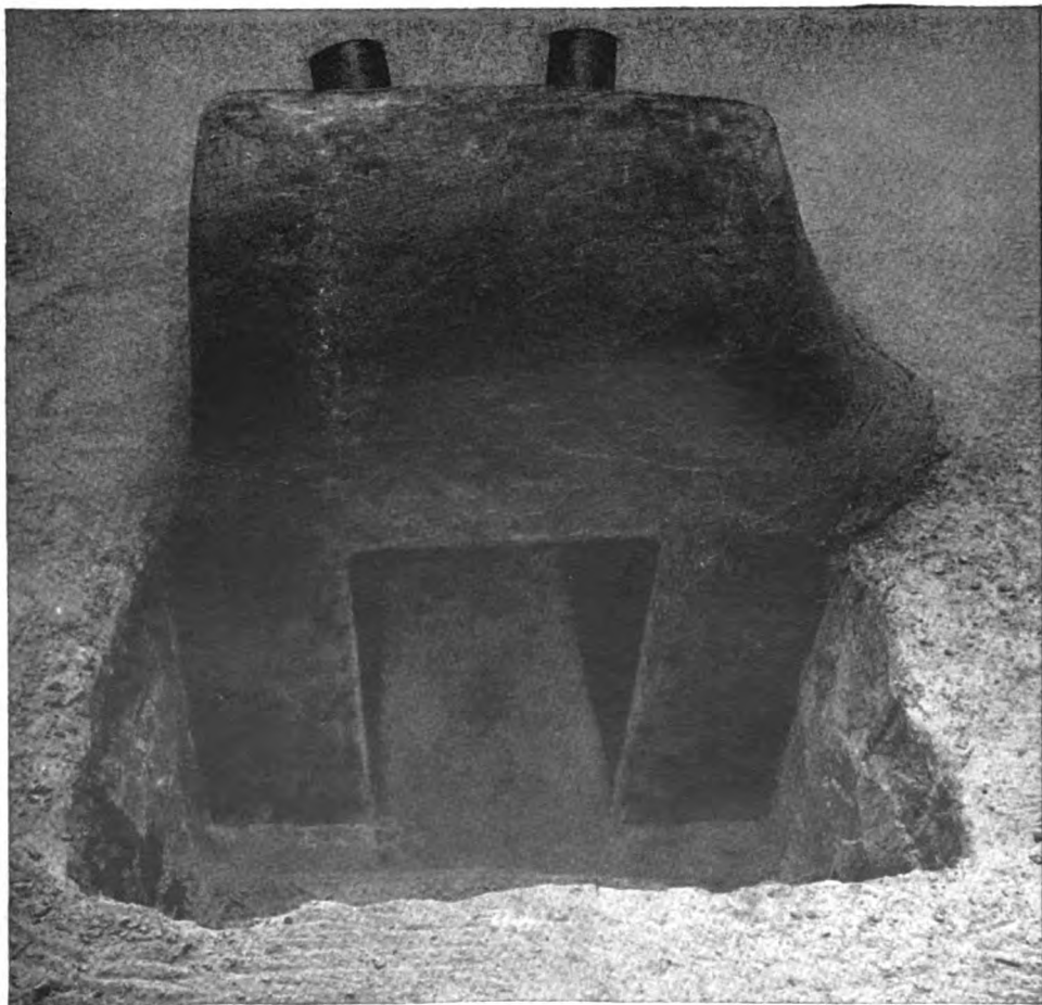
Figure 81. Oil drum oven, side view.
