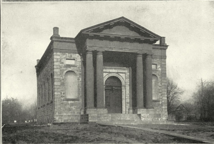
OLD CHAPEL ON OLD SITE (above) ON PRESENT SITE NEAR CEMETERY (below)
