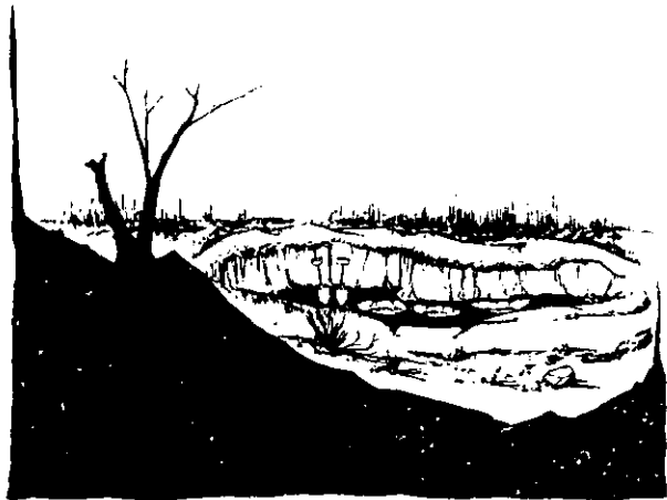
Figure D-1. Emplacement after excavation of all loose earth.
