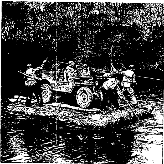
Figure 19. Expedient ferry using brush-filled canvas.
