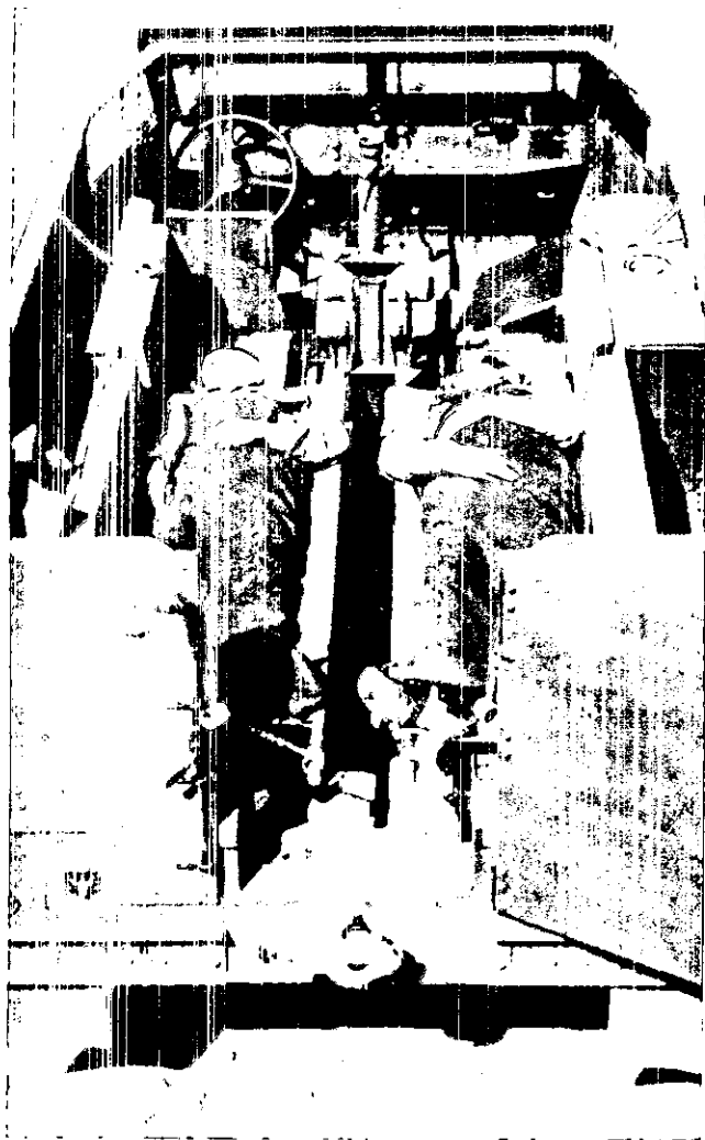
Figure 186. Half-track converted for patient carrier.
