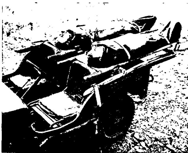
Figure 172. Two litters loaded on improvised sapling frame.
