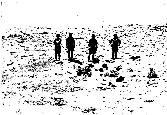
FIGURE-57.—In front of the men is a vehicle, dug in and camouflaged to blend with the background. Spoil is slightly mounded around the excavation and gradually sloped to meet existing terrain level. Both vehicle and spoil are covered with a light screen made of chicken wire and cloth, over which is spread sand, a few rocks, and some brush.
