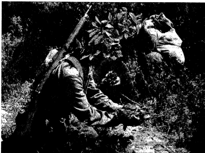
FIGURE 10.—Short exposed stretches of infrequently used access routes may be obliterated by placing brush over a scarred area or by brushing leaves, dirt, or other debris over it.
