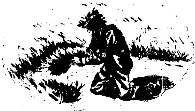
FIGURE 39.—If time permits, place sod or brush over new spoil. Sod must be watered to keep it alive.
