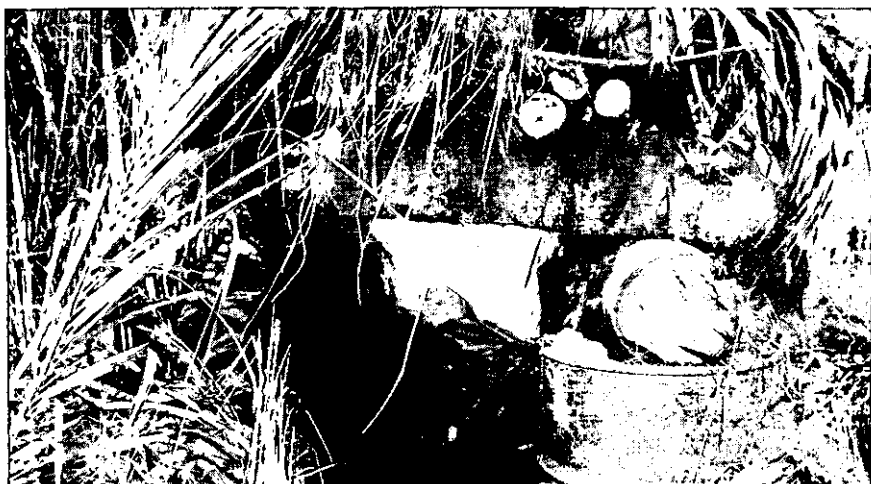
FIGURE 89.—Entrance to firing position concealed in jungle. Natural materials arranged over entrance and loop-holes would make position difficult to see at close range.
