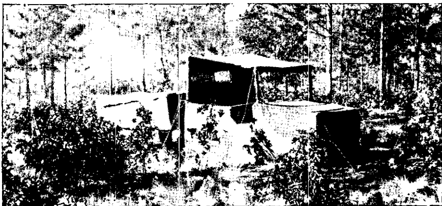
FIGURE 79.—Decoy truck made of frame covered with cloth.
