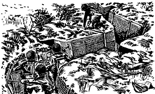
Figure 12. Installing burlap and chicken-wire revetment.
