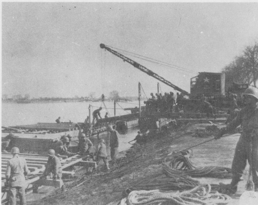
Photo No. 17 HEAVY PONTON BRIDGE UNDER CONSTRUCTION AT NIERSTEIN.
