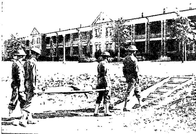
FIGURE 101.—Upstairs carry, third step.
