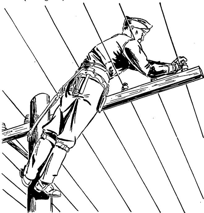
Figure 52. Working on outer wire of cross arm.
